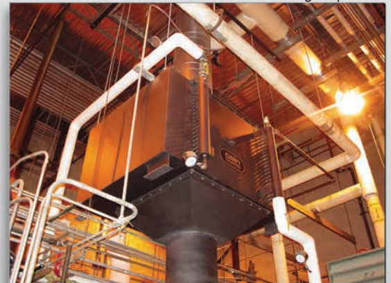
Installation: ceiling suspension
