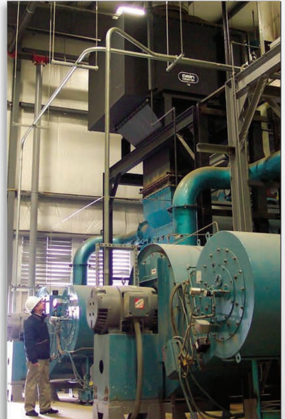
Installation: structural support stand
