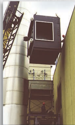
Brewery, Ontario, Canada (1) RTR-1V2Q28CSS recovering Btu from (1) 95,000 pph steam boiler; Reducing 505°F @ 24278 SCFM to 333°F; Raising 196 gpm boiler feedwater entering at 225°F to 278°F.
