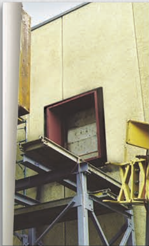
Brewery, Ontario, Canada (1) RTR-1V2Q28CSS recovering Btu from (1) 95,000 pph steam boiler; Reducing 505°F @ 24278 SCFM to 333°F; Raising 196 gpm boiler feedwater entering at 225°F to 278°F.
